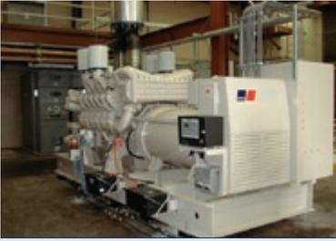
MTU Onsite Energy standby power systems installed at Fairfax County wastewater pumping stations operate at 1,800 rpm, or twice the speed of the units they replaced. The new generators also feature state-of-the-art electronics and will start and accept load within 10 seconds.
